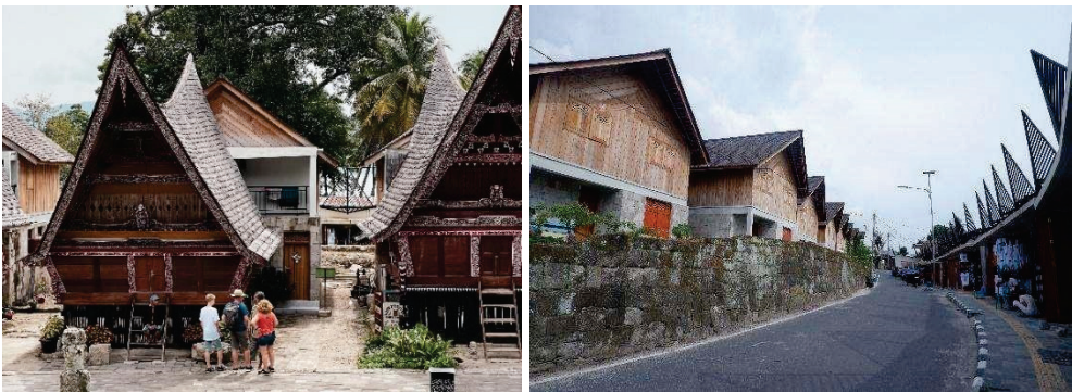
Figure 5. Traditional house extension from inside and outside perspective
